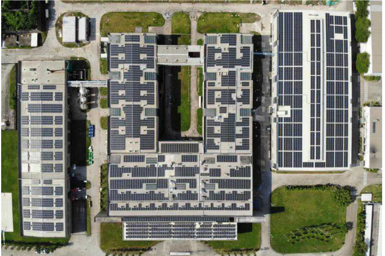
Solar panels have been installed on all roofs of ECCO Tannery Xiamen since 2019
